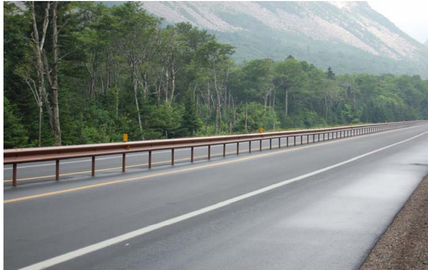
Nu-Guard-31™ Double-Faced Median, Galvanized & Powder Coated, New Hampshire
