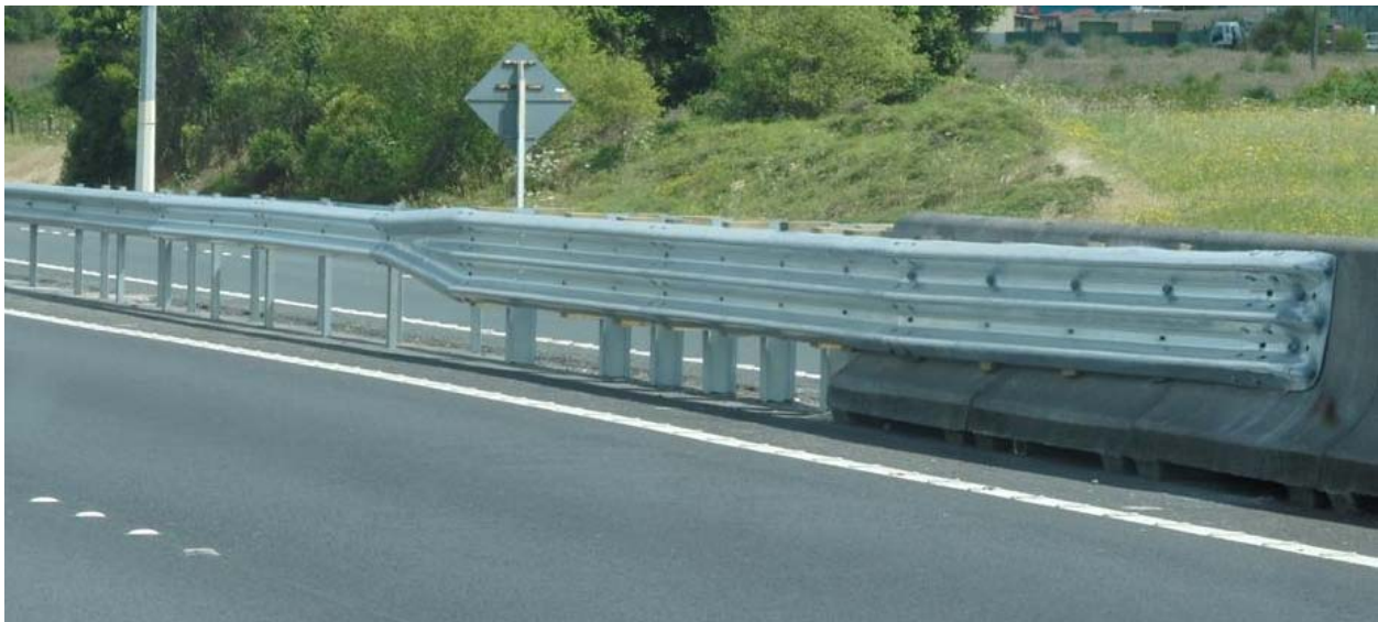
Nu-Guard-31™ Transition To A Thrie-Beam Bridge Connection
